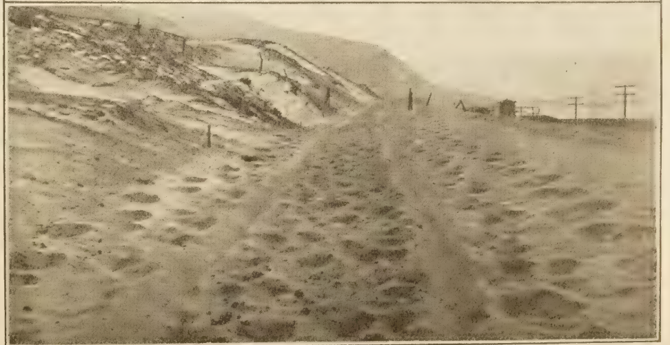
USE OF OIL ON ROADS TO CONTROL SHIFTING SAND. TOP—THE EFFECT OF WIND ACTION ON UNPROTECTED FILL SLOPES AT BLALOCK, IN GILLIAM COUNTY, OREG., ON FEDERAL-AID PROJECT NO. 24. CENTER—NEWLY GRADED SECTION OF FEDERAL-AID PROJECT NO. 37, NEAR CELILO, WASCO COUNTY, OREG., COVERED WITH STRAW AND STABLE MANURE. BOTTOM—NEWLY GRADED SECTION OF FEDERAL-AID PROJECT NO. 25, AT SHERMAN, OREG., BEFORE OILING. NOTE THE DEEP RUTS THROUGH THE SAND. IN THE UPPER LEFT OF THE PICTURE IS SHOWN A PORTION OF THE SAND HILL WHICH WAS OILED BY THE RAILROAD COMPANY.
